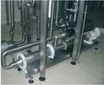
PCM Moineau™ Hygienic Progressing Cavity pump for yogurt transfer.
